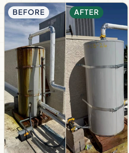
Rooftop water heater replacement
